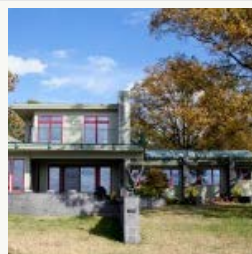
An exquisite restoration of the mid-century Modern Lafayette River Residence by Pentecost Deal & Associates. Photo by Lauren L. Keim.
